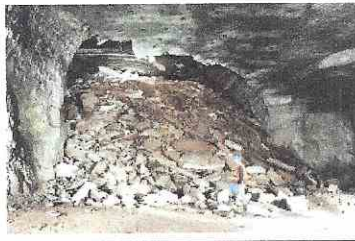
Notice Rock Bolts Ceiling and rock strata
